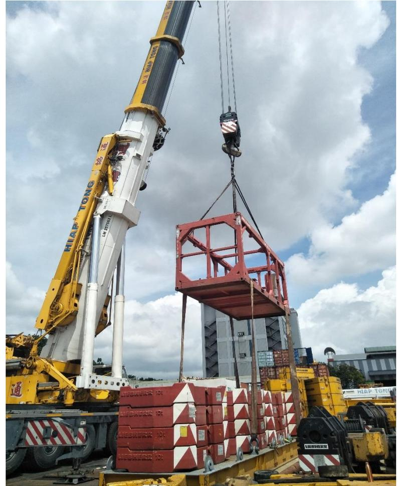
**LOAD TEST ON SKID**
